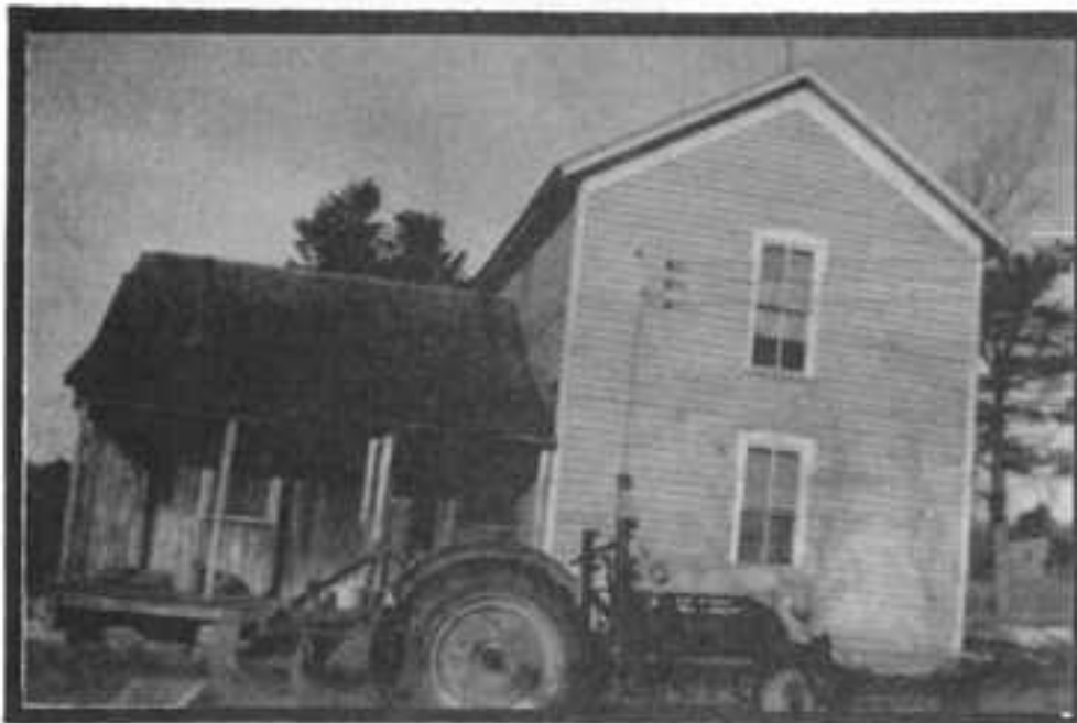
(above) photocopy of the 1899 deed transferring ownership of property containing one hundred acres from Manasseh Catron to his son, Jacob and (left) a 1949 photograph of the home he built there. Note the wellhead through the porch and the well bucket hanging from the post.
